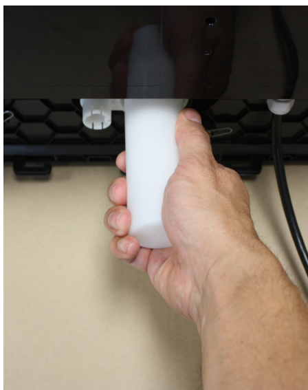
Figure 17: Condensate trap installation
