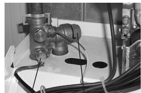
C.H. sensor Safety valve
