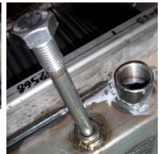
threaded bar that must be unscrewed and taken out in order to allow the draining of the water from the boiler
