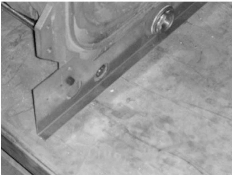
5.1.19. Fit casing lower support in position as shown using the hex head screws supplied.
