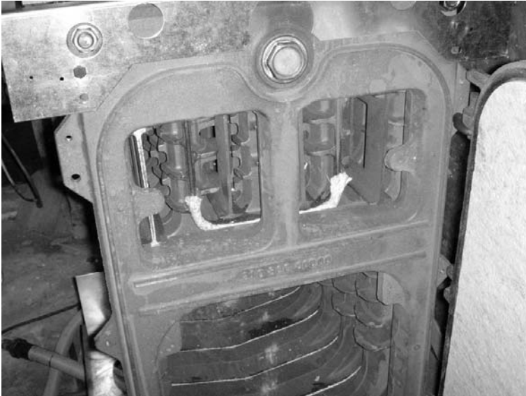
5.1.20. Pictorial view of divider plate in position and casing upper stiffener fitted.
