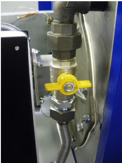
Figure 7.2.1 - Gas Isolating Valve (97 & 116 shown)
