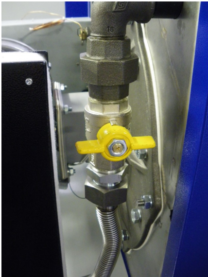
Figure 8.1.1 - Gas Isolating Valve
