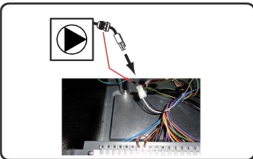
3. Use one of the spare holes in the bottom plate of the boiler to assemble the cable gland and pump signal cable.
