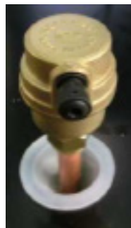
AERATOR - LOCATED ON TOP OF BOILER
