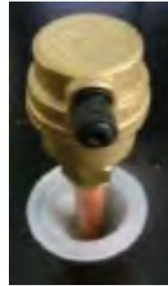
AERATOR - LOCATED ON TOP OF BOILER
