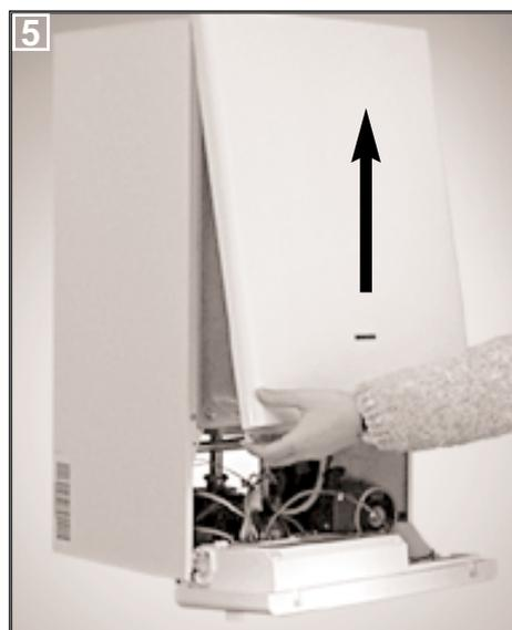
To dismantle the front casing panel it is necessary to:
