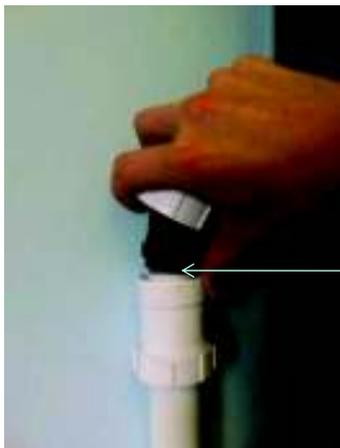
Locate elbow over inner connection and tighten nut.
