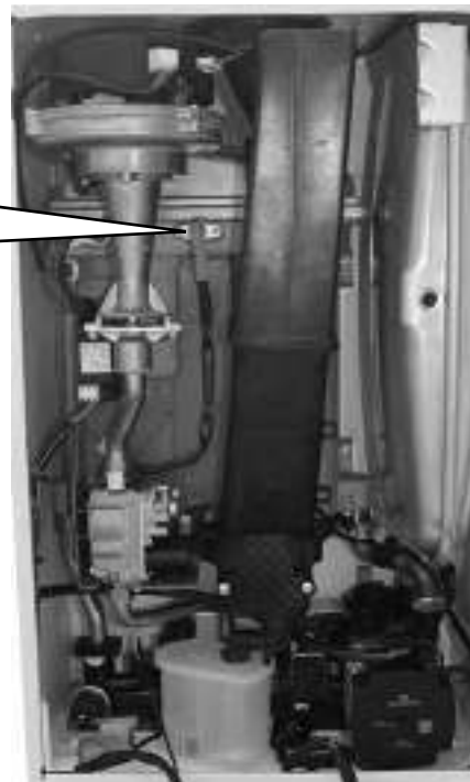
Flame Detection Electrode
