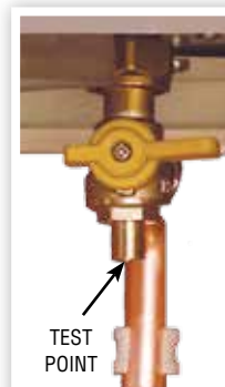
FIGURE 23. GAS PRESSURE TEST POINT
